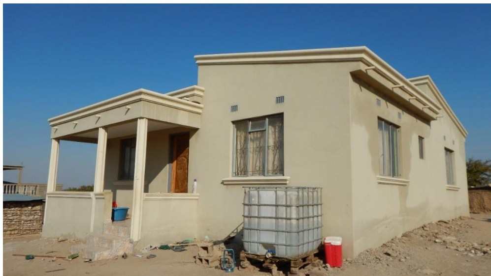
Figure 4. House with water catchment system constructed in 2011 using conventional building materials, glass windows, and wood door.
