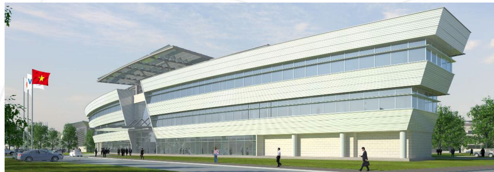
Management Center and S/C Control Center
