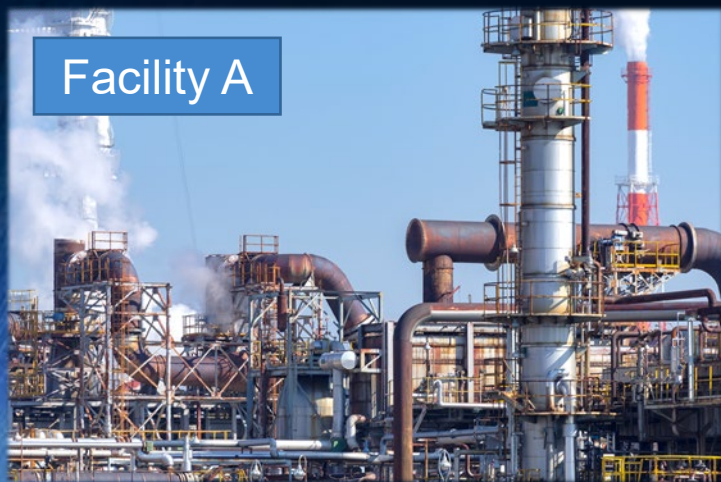
Oil combustion facility
