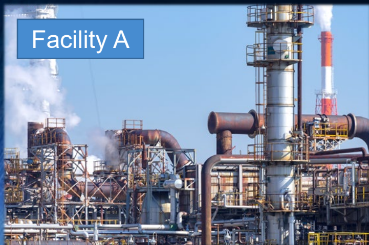
Oil combustion facility
